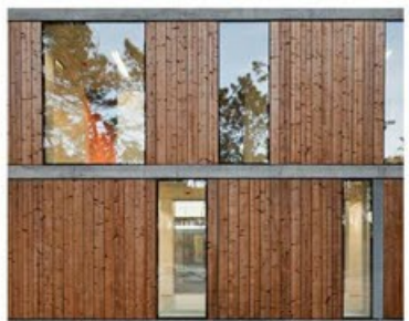
Timber effect cladding with shadow gap
