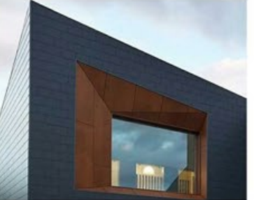
Dark grey cladding with timber effect panels
